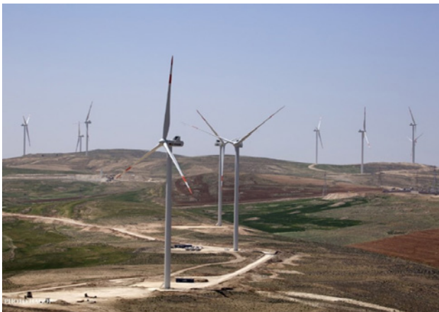
UfM-labelled project Tafila Wind Farm
