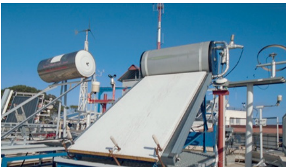
Figure 15: CDER - LEsS Lab in Algeria
