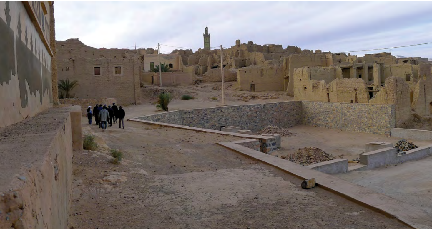
An abandoned part of the historic Ksar in Figuig.
